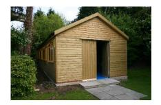
We strongly advise a single course of semi-engineering bricks to place your garage on as it helps keep moisture out of the building. If the building is to be placed directly onto a concrete based this will affect the warranty of the building and we can't be held liable for any water ingress or up take.
